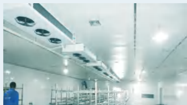
Cold Storage Installation Picture
