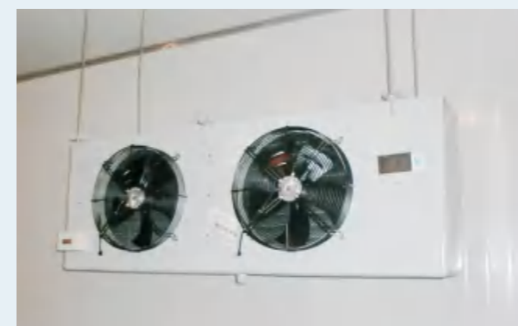
Air Cooler Installation Picture
