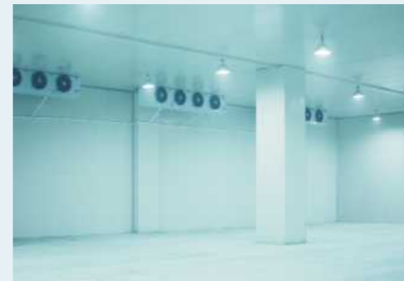
Air Cooler Installation Picture
