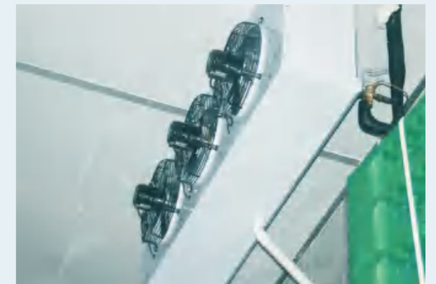
Air Cooler Installation Picture
