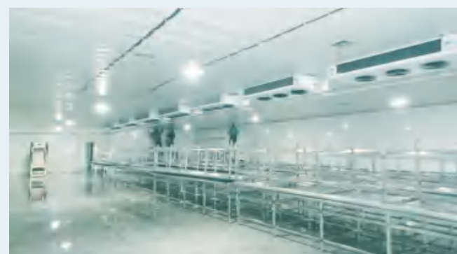
Cold Storage Installation Picture
