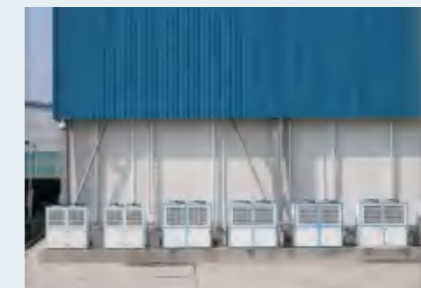
Finished Condensing Unit Installation
