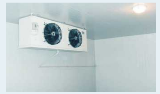
Air Cooler Installation Picture
